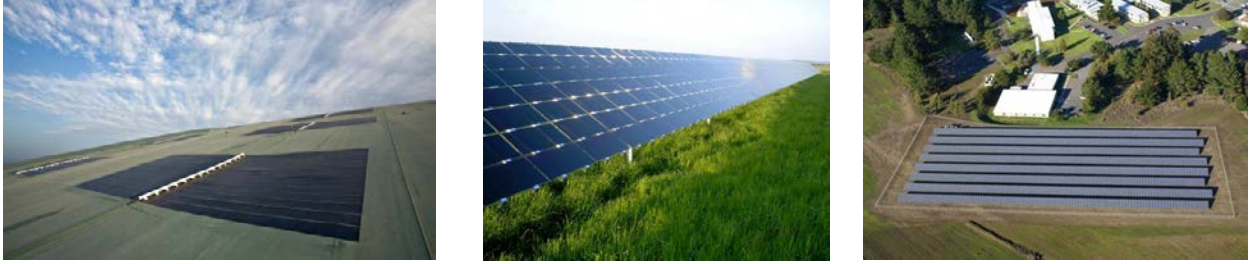
Figure 6. Thin-film solar panels installed on (left) solar energy cover and (middle/right) fixed-tilt mounting system. Photos from (left) Republic Services, Inc., NREL 23817, (middle) Beck Energy, NREL 14726, and (right) U.S. Coast Guard Petaluma Site, NREL 17395
