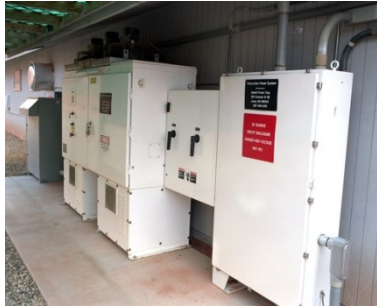
Figure 7. String inverter. Photo by Warren Gretz, NREL 07985
